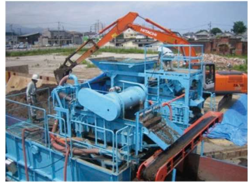
Heavy Metal Soil Washing Equipment
