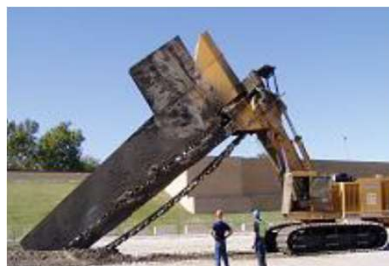
Barrier application by trench
